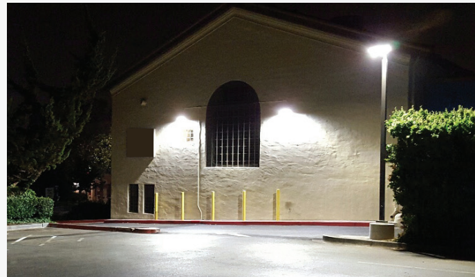
LED Lighting Upgrade
